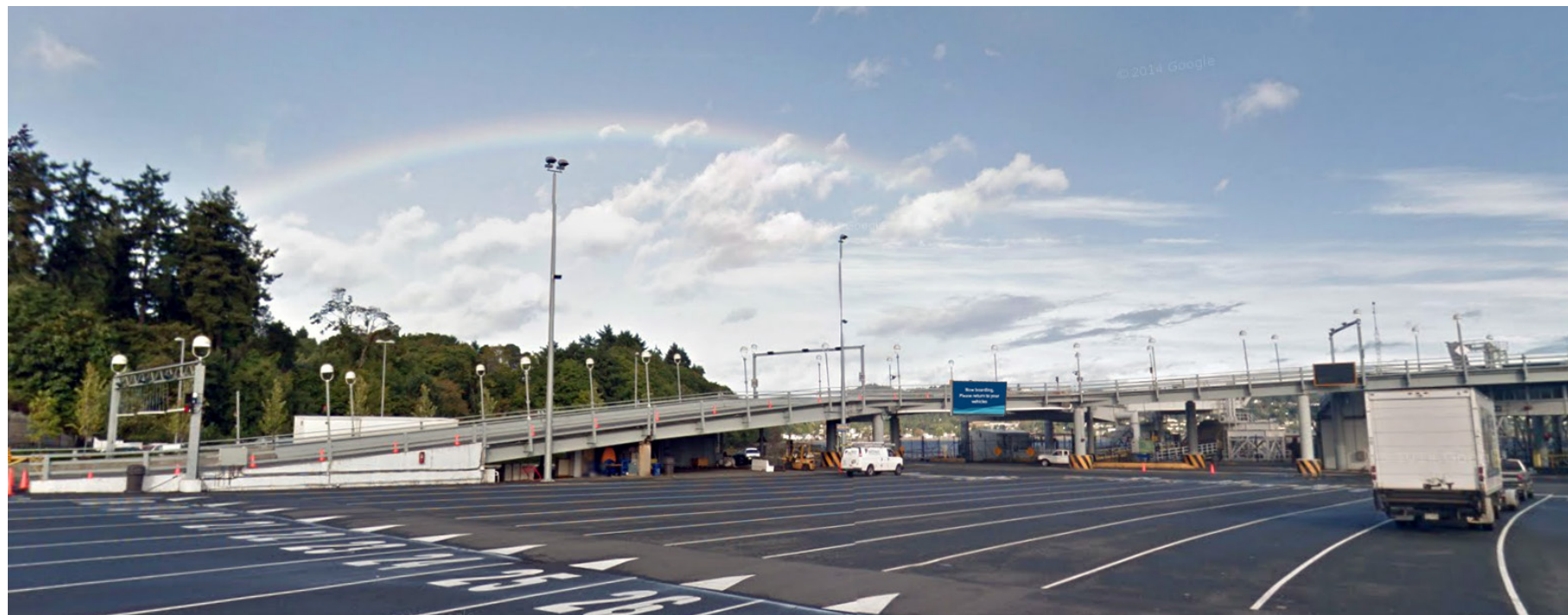
SIGN A : VIEW 3 Taken from vehicle in lane 29 in front of ramp
